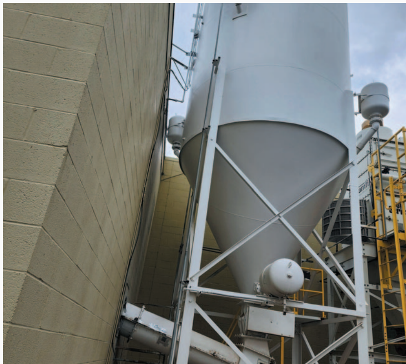
Global Manufacturing air blasters on a dust reclamation silo, which allows the customer to reuse the material in the production process.
