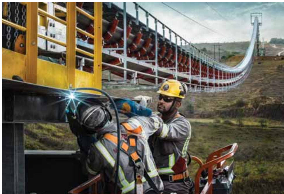
The Flyingbelt is suspended on four track ropes, standing on a ropeway 7.2km long and up to 36m high.
