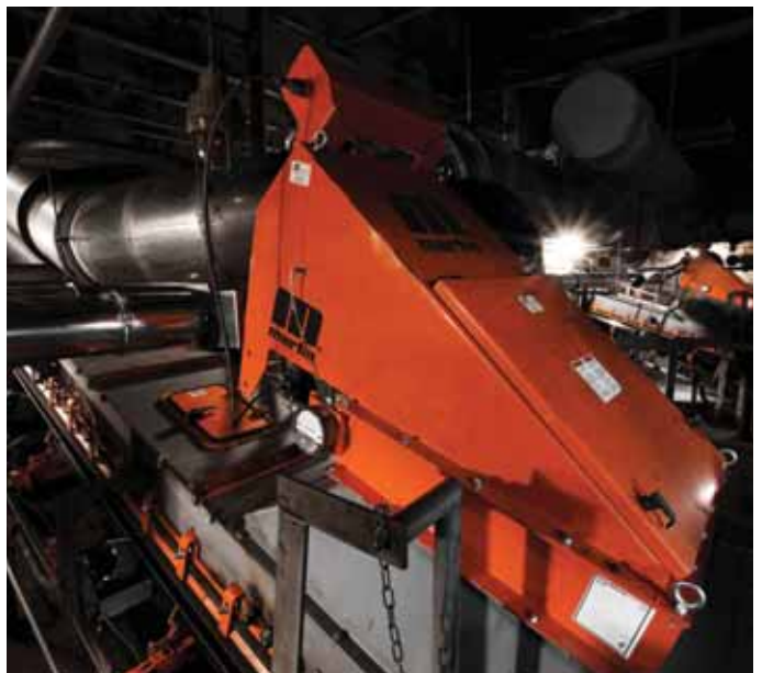
Insertable air cleaners filter dust-bearing air at the source, without the ductwork or large fans of central collection systems.
