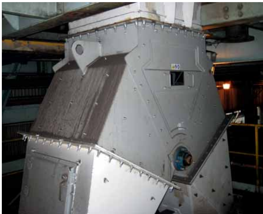
Vortex diverter valves feature removable blades, replaceable abrasion-resistant liners, and easy access panels to allow in-line inspection, maintenance, repair or replacement.
