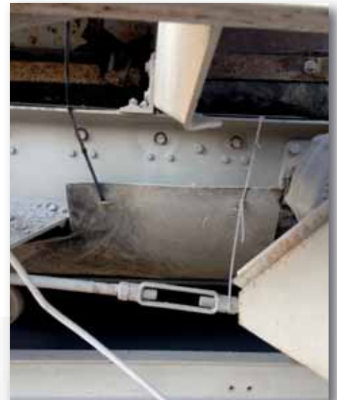
One of the most important jobs of the load point is to provide a seal that prevents material spillage and controls dust. In this photo, spillage and dust are likely because a proper seal has not been achieved.
