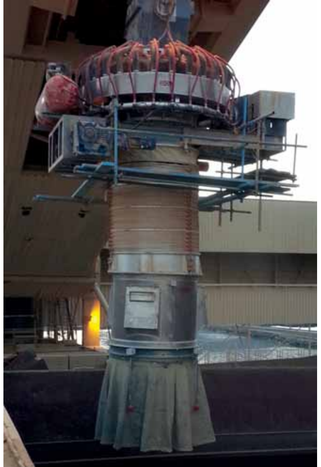
Loading out equipment installation complete.
