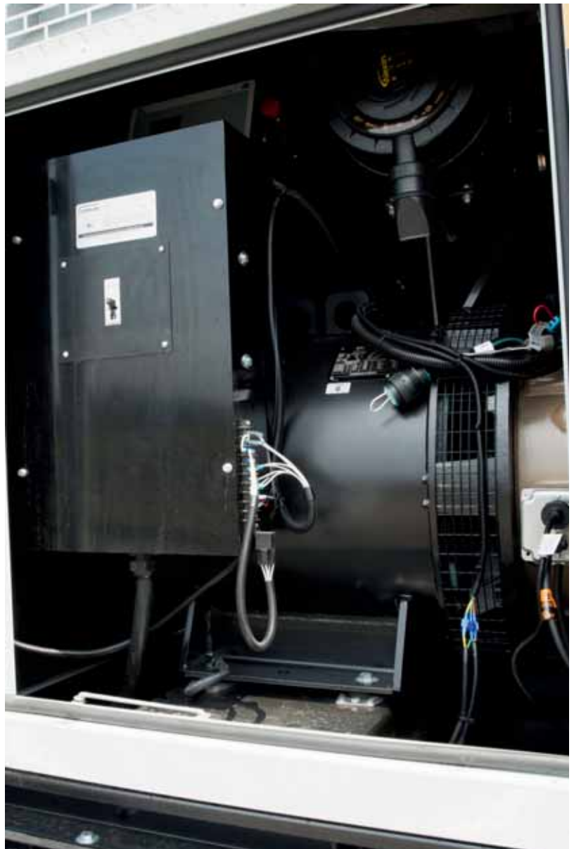
The unit is powered by a 480V/150KW generator with a 6.8 litre John Deere Tier III flex diesel engine.
