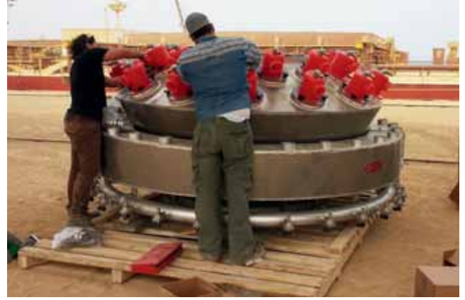
Pre-installation assembly of compact filter module cartridges.
