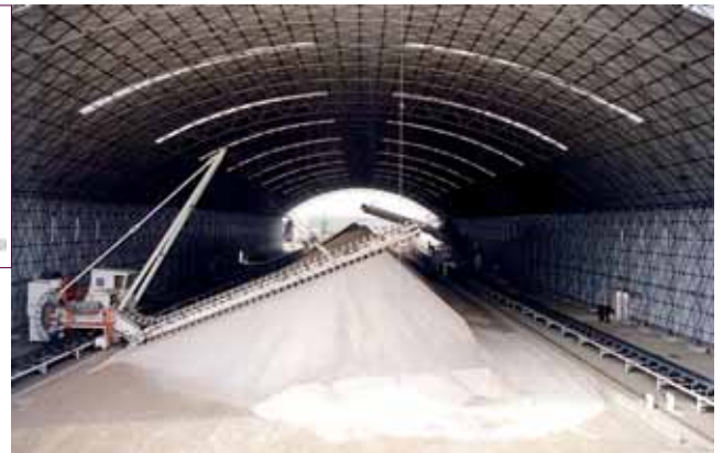
Bent: This is selected when the footprint space is very constrained. Above, bent profile. Right, raw material storage in Chile.
