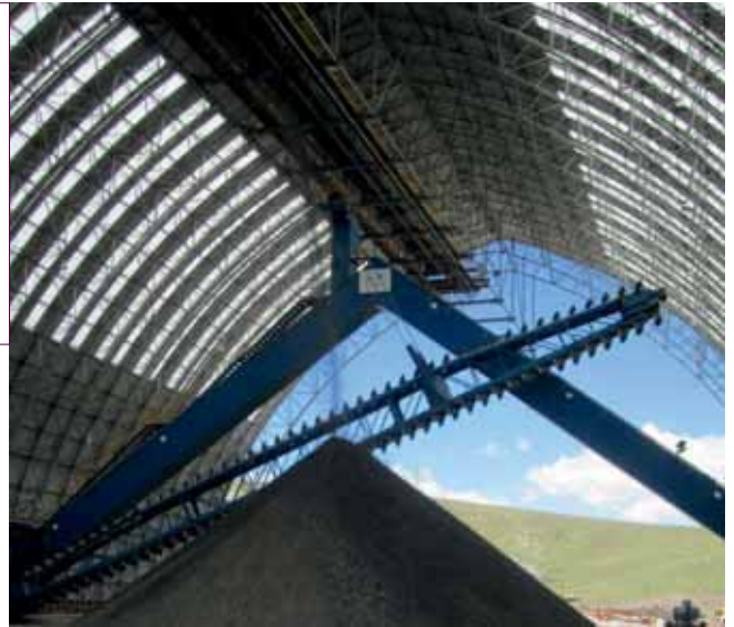
Acute: This geometry is designed to carry concentrated loads such as walkways or tripper cars, and to shed snow. Above, acute profile. Right, mineral ore storage in Peru.
