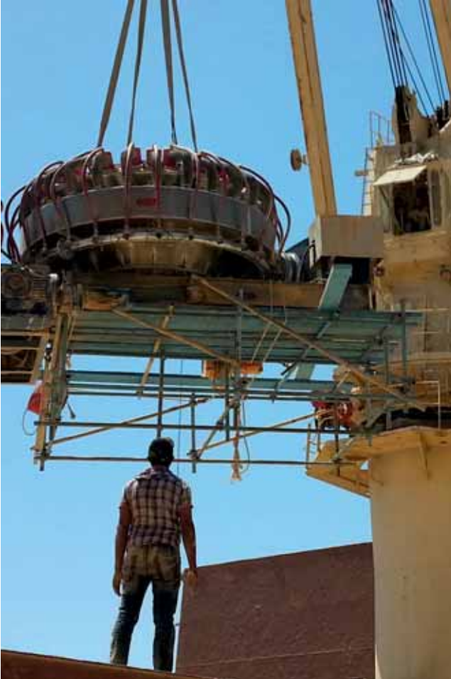
Compact filter module being hoisted into position.
