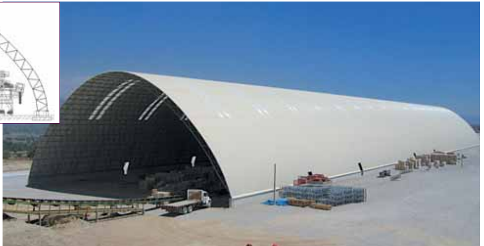
Compound curve: Alternative to 'Bent' when space is constrained. Above, compound curve profile. Right, coal and limestone storage in Mexico.
