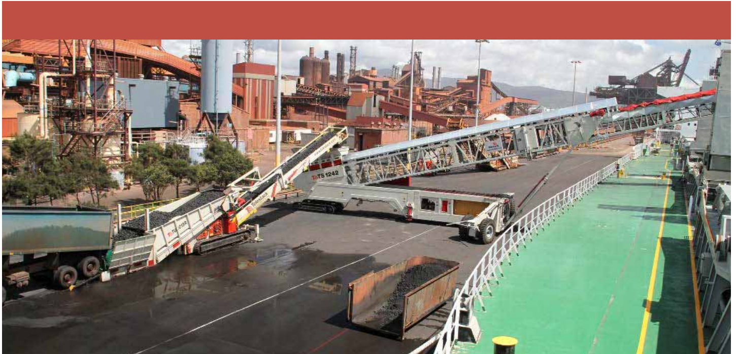
Radial Telescopic Shiploader and Mobile Truck Unloader loading pet coke to Handymax vessels
