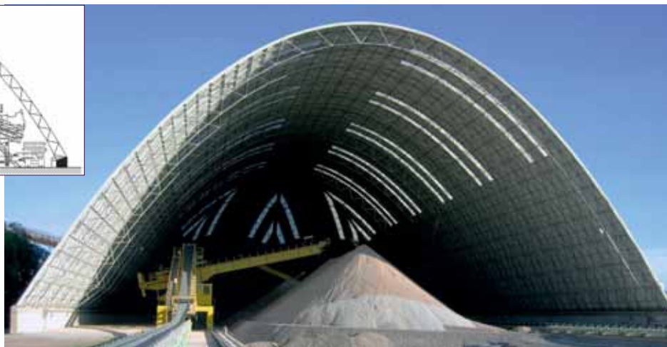
Parabolic: These work best for the longest spans with heavy gravity loads such as snow, and moderate wind loads. Above, parabolic profile. Right, limestone storage in Mexico.
