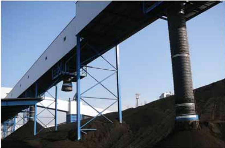
Stockpile coal loading spout, power plant Ledvice, Czech Republic
