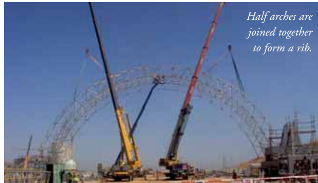
Half arches are pre-assembled on a project in Tunisia.
