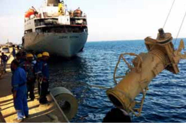
Removal of existing unsatisfactory loading spout.
