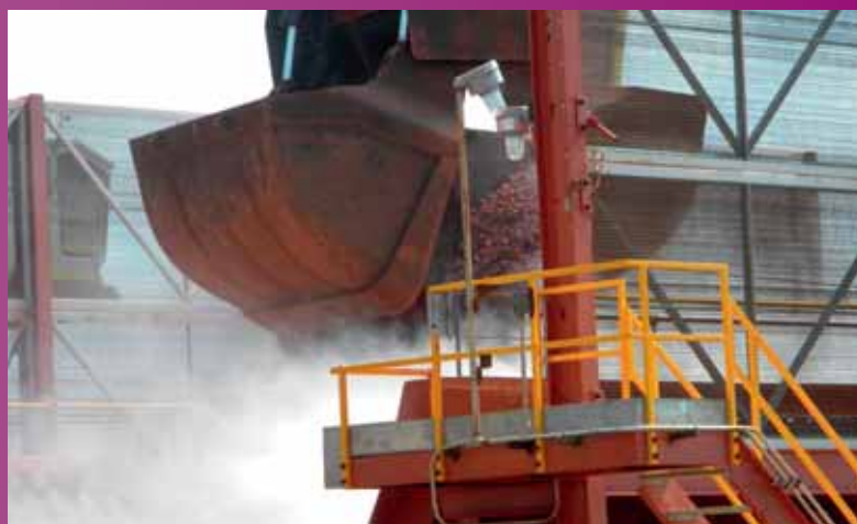
Dry Fog prevents fugitive dust from escaping hopper during unloading. (Material: bauxite.)
