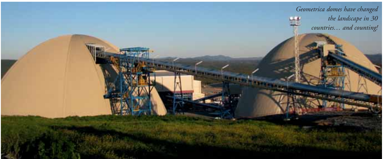
A multitude of raw materials, from limestone to clinker to coal, are safely enclosed under Geometrica domes.
