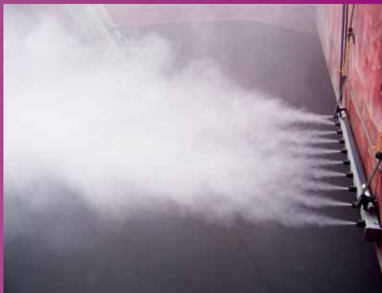
Dry Fog manifold which fills the open barge with fog and prevents dust from escaping the hatch during the loading process. (Material – cement.)
