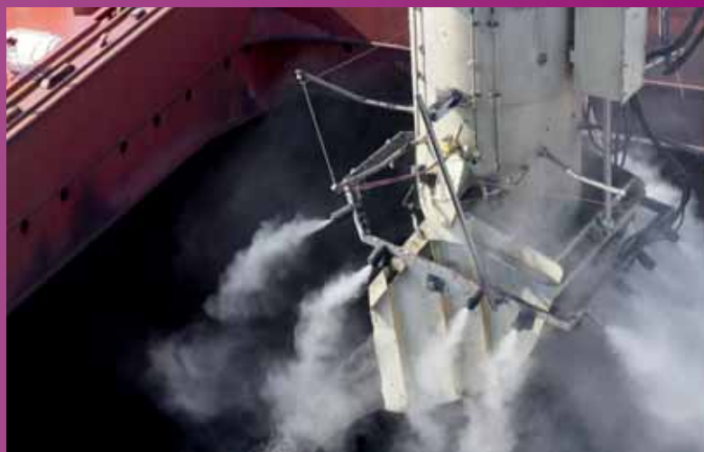
A Dry Fog ring custom designed and engineered for the loading chute. Higher capacity ultrasonic nozzles and custom nozzle adaptors provide operators with the flexibility to provide a stronger fog that covers a larger area and distance of the ship's hatch. (Material: coal.)
