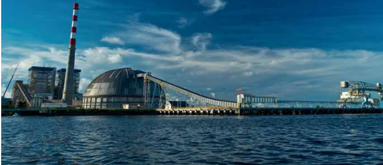
Pupuk Kaltim Dome, 81m Coal boiler plant, Pupuk Kaltim, Bontang, Kalimantan Timur, Indonesia
