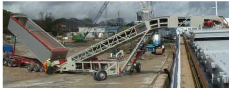
Cambered boom Shiploader loading coaster vessel direct from Trucks
