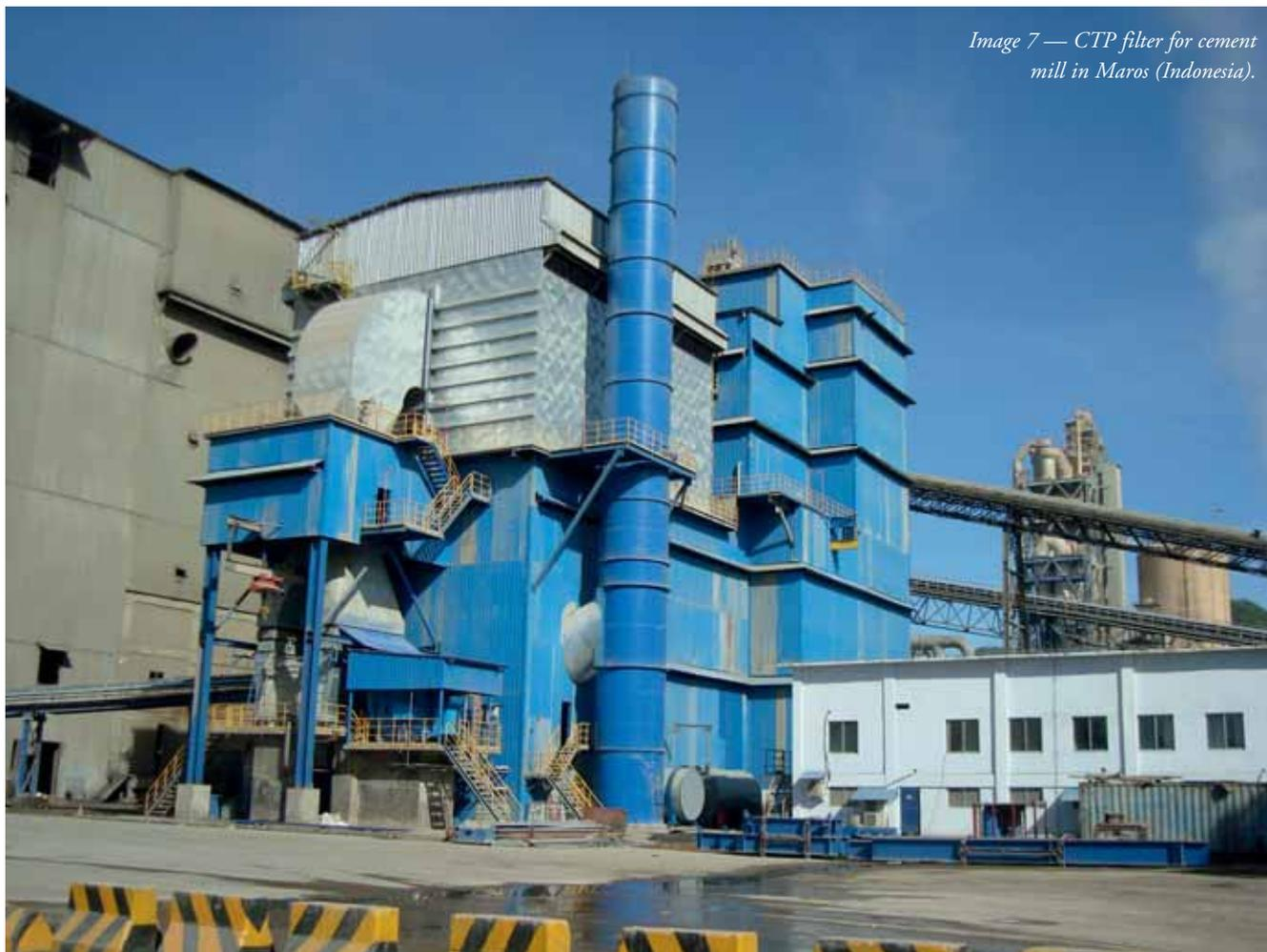
**Project:** clinker cooler bag filter for kiln line 1 & 2 — 7.5m bag length - capacity 750,000Am<sup>3</sup>/h.
