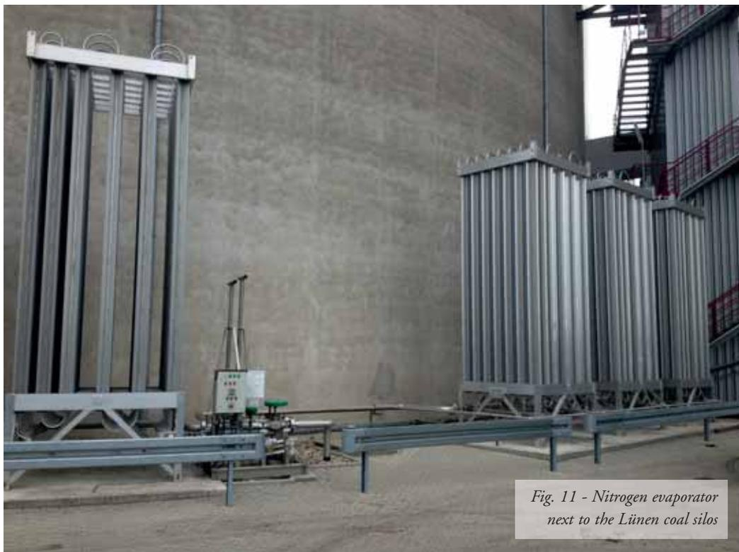
Fig. 11 - Nitrogen evaporator next to the Lünen coal silos
