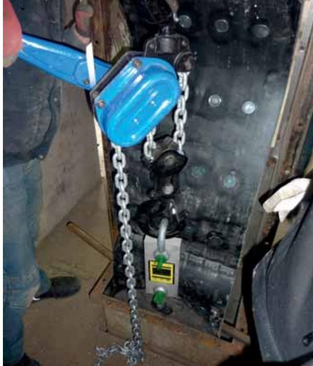
then installed and tensioned using belt clamps and a tension meter.
