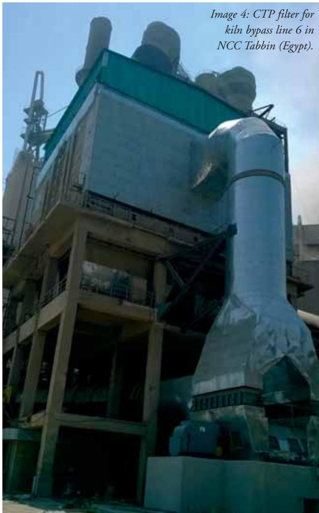
Image 4: CTP filter for kiln bypass line 6 in NCC Tabbin (Egypt).
