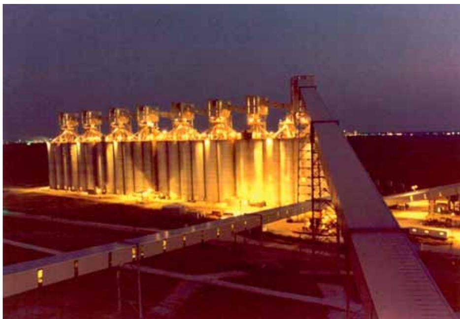
thin layer of air supports both the carrying and return sides of the belt.
