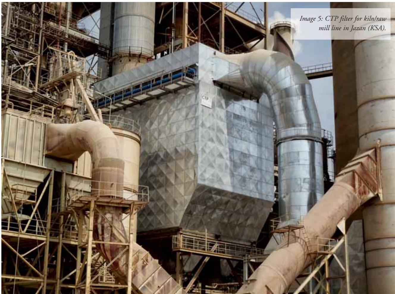
900,000Am<sup>3</sup>/h and clinker cooler bag filter — 8m bag length — capacity 600,000Am<sup>3</sup>/h for new 5,000tpd kiln line.
