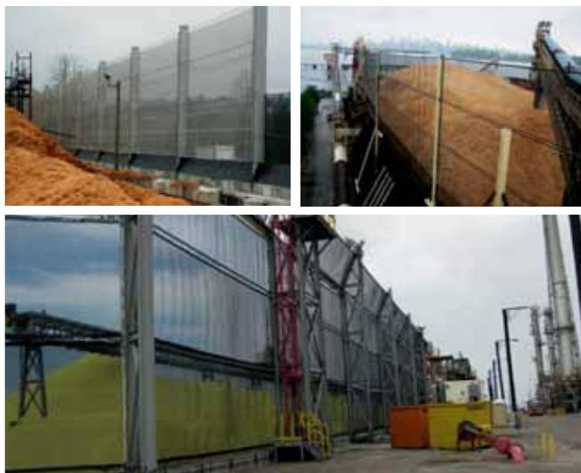
access requirements. All of WeatherSolve's fences are custom designed to suit the individual needs of the customer. The company is able to accommodate conveyors or any other equipment, doorways and gates for people or vehicles. It also has retractable systems for areas requiring regular access.
