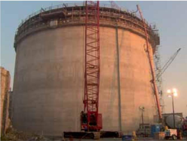
simultaneously or where blending different grades of the same commodity is desired. Properly designed and constructed concrete silos have a very long life-span, and the concrete also acts as an insulator, protecting the grain inside from potential condensation that may result from daily ambient temperature changes.
