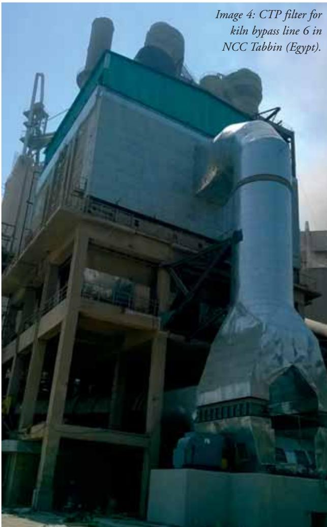
Image 4: CTP filter for kiln bypass line 6 in NCC Tabbin (Egypt).
