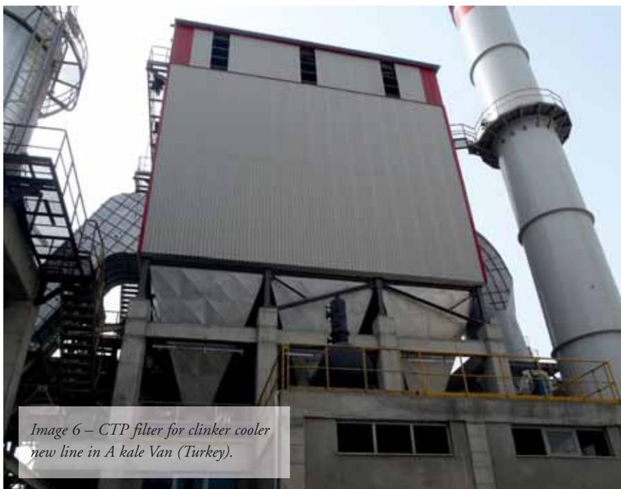
Image 6 – CTP filter for clinker cooler new line in A kale Van (Turkey).
