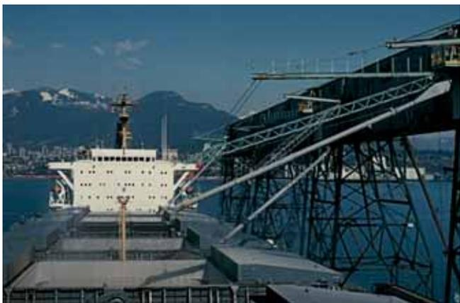
Berth 2 at the Pacific Elevators grain export terminal was upgraded to accommodate and load larger bulk carriers up to 50,000dwt.
