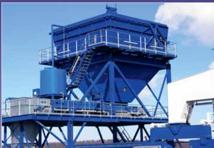
Hopper cars for ship unloading
