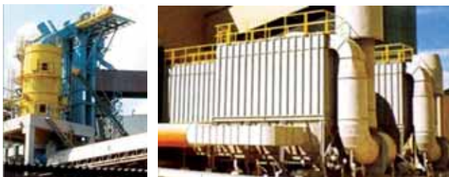
Fig.4. Rectangular and round filters in centralized systems aspirating several machines.
