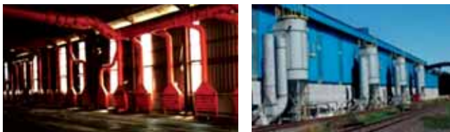
Fig 8. Railcar reception with lateral dust collectors alongside the unloading area and filters.
