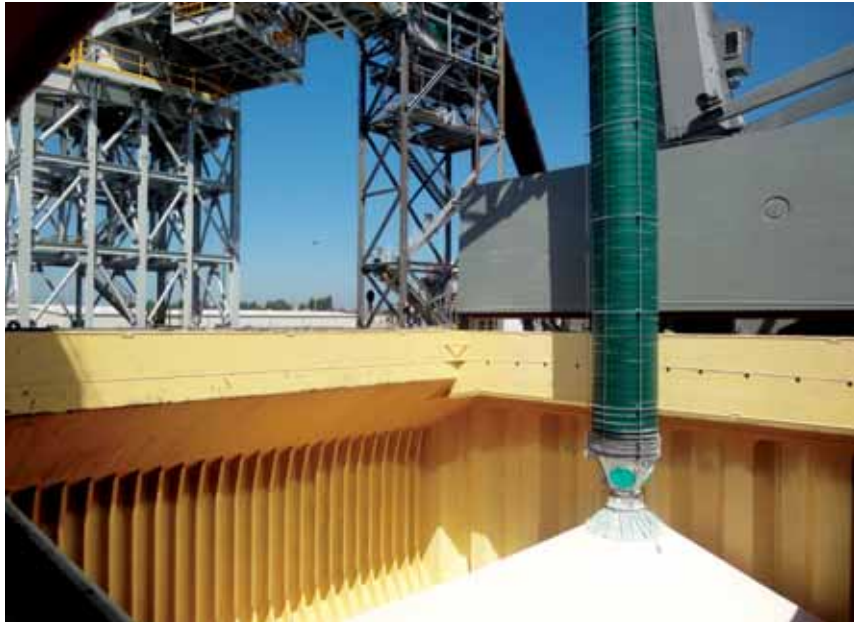
Dust-free soda ash loading at rates of up to 2,000tph (tonnes per hour) at Port of Portland, Oregon, USA.
