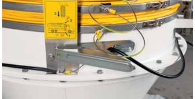
Chute outlet with earth connection according to ATEX directive.
