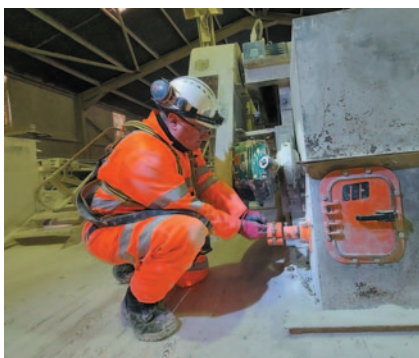
Copyright © Martin Engineering 2025. Installing remote monitoring for belt cleaners significantly reduces physical visits to each conveyor.
