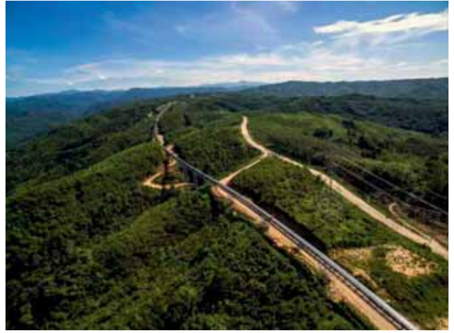
The route of the overland conveyor for the end customer, Cemindo Gemilang, passes through the middle of the rain forest.
