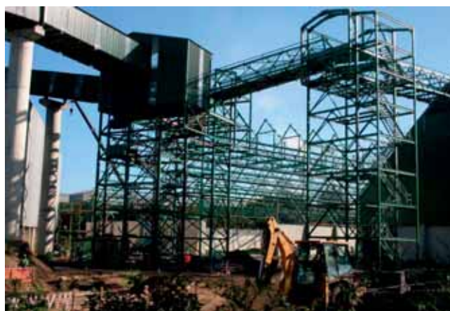
Construction of conveyors and transfer house at the Richards Bay multi product terminal, KwaZulu-Natal, South Africa.
