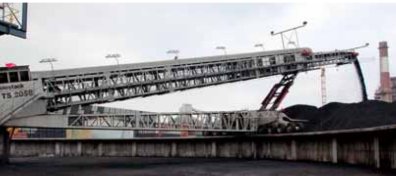
Radial telescopic stockpiling coal @ 2000tph in powerplant receiving from ship unloading system
