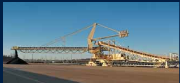
Coal Stockyard with Pylon-type Stacker
