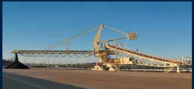
Coal Stockyard with Pylon-type Stacker
