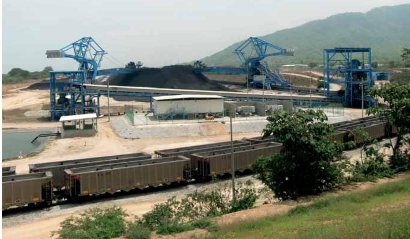
Complete Sandvik stockyard system for an coal export terminal in Colombia.
