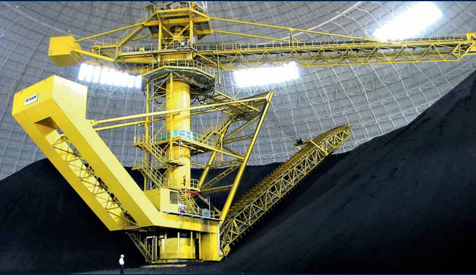
Circular Stockyard with Cantilever Reclaimer
