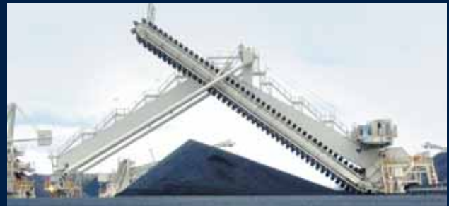
Portal Scraper Reclaimer with Twin-Boom
