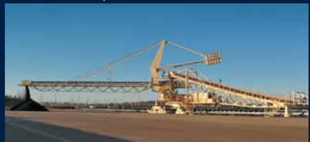
Coal Stockyard with Pylon-type Stacker
