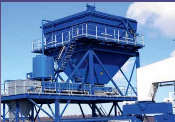
Hopper cars for ship unloading
