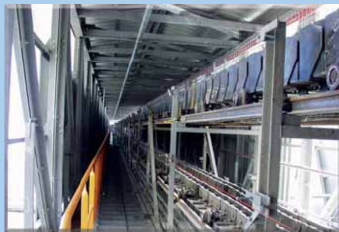
Clinker pan conveyor
