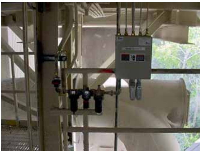
The air cannons in the main production line network are equipped with a negative pressure-firing valve design that delivers reliable operation and long service life in challenging applications.
