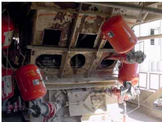
In order to prevent reduced flow and blockages at the Ash Grove Louisville plant, Martin Engineering installed a network of 25 air cannons to remove material that becomes adhered to vessel walls.
