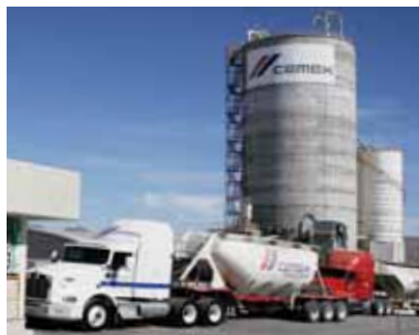
Cement import terminal for CEMEX, Mexico
