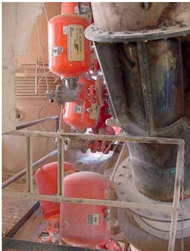
The air cannons were installed during a scheduled maintenance outage, starting below the riser orifice, as the duct reduces in size to increase velocity.
