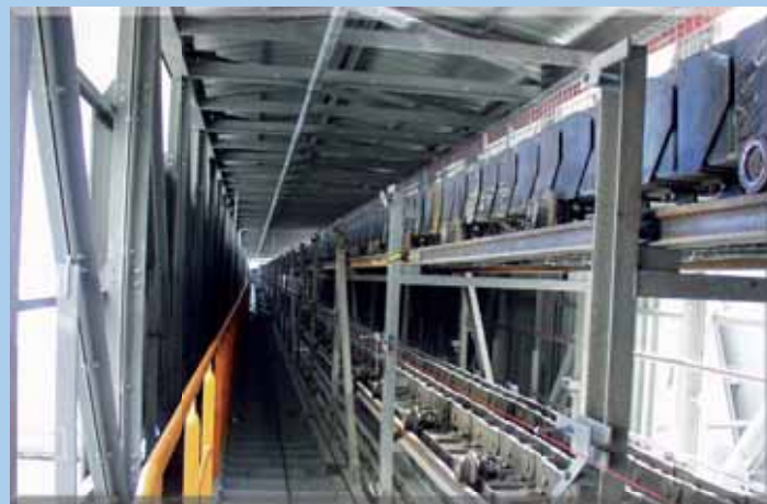
Clinker pan conveyor
