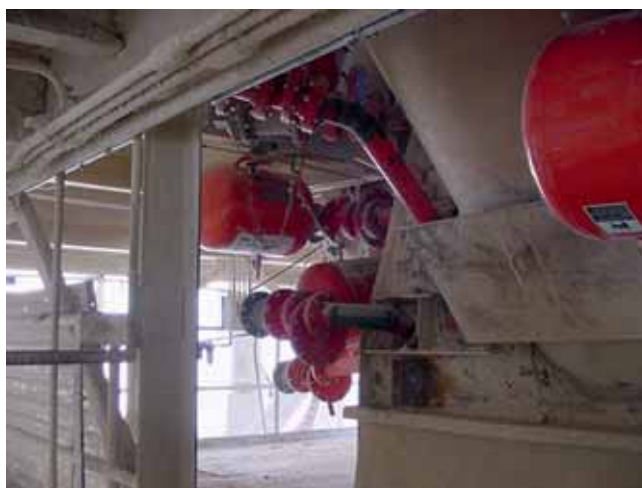
A crew from Martin Services installed the entire system, including cannons, air lines and controls, as well as the company's Thermo Shields™ on each unit.
