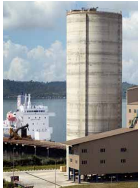
Marine Cement Terminal for Cement Industries (Sabah) Lahad Datu, Malaysia
