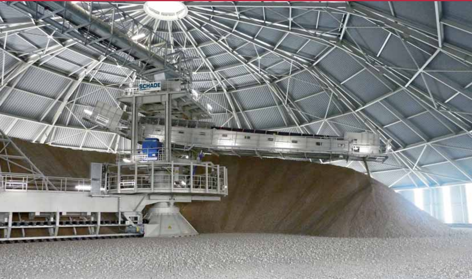
Circular Bridge Stacker/Scrapper Reclaimer, Limestone
