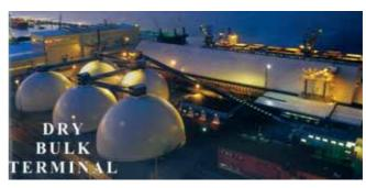
includes three new dome storage silos (total additional storage of 27,400 tonnes) plus associated intake and outloading belt conveyor systems. Completion is scheduled for June 2013.
