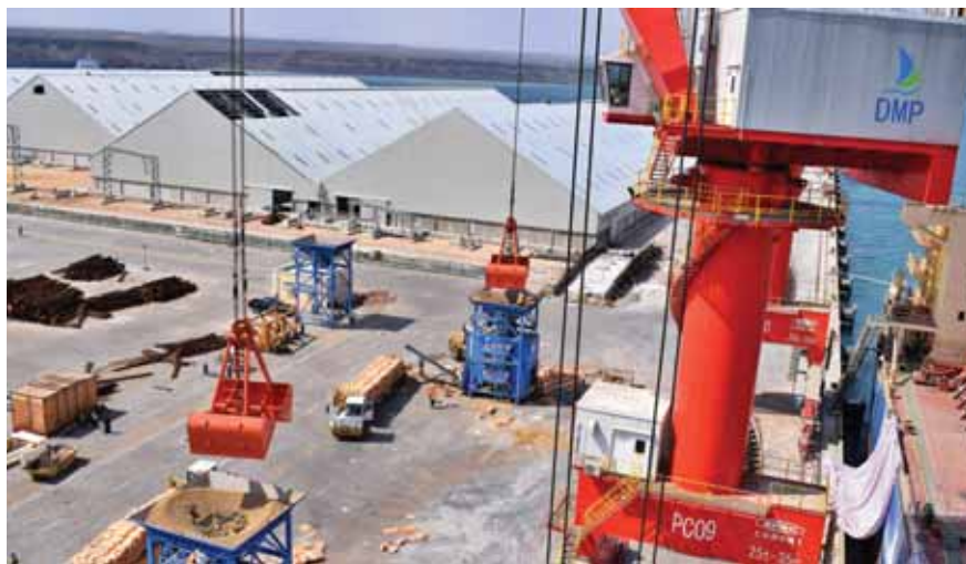
Rapidpack port operations, Mobile Bagging Machines and grabs at DMP.
