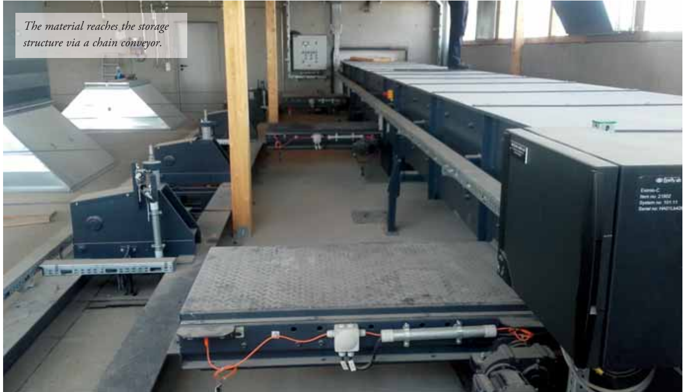
The disc screen removes wood pieces that are too long. The sorted excess lengths go straight to a container.
