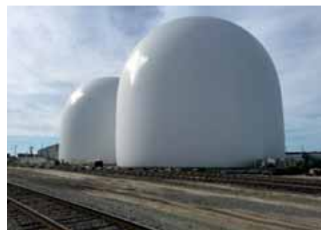
Enviva's 17-storey wood pellet storage domes at the Port of Wilmington will commence exports in the second half of 2016.
