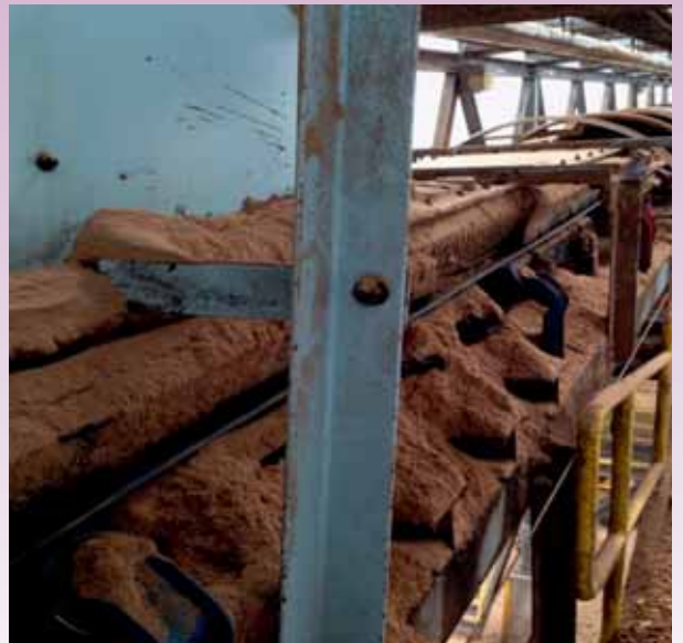
BEFORE: Fugitive material build up on the conveyor chute and the load zone area caused by chute holes and improper sealing systems.
