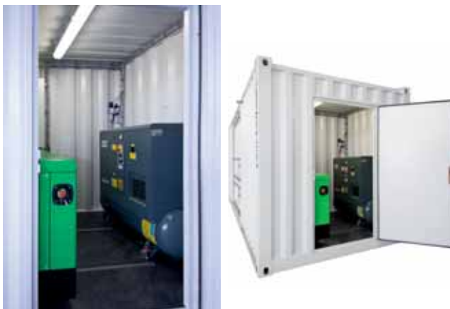
Bottom container with diesel generator and compressor for instrument air.
