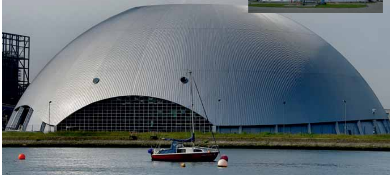
Marchwood Energy Facility, Southampton, UK with (inset) a clear view of the dome's sweeping skirt.
