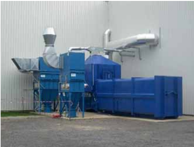
Image 2: The two explosion rated PowerCore dust collectors for paper dust at ASFI in the Czech Republic are characterized by their long filter life, low maintenance and compact design.
