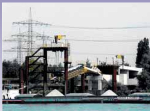
Ship loading systems
