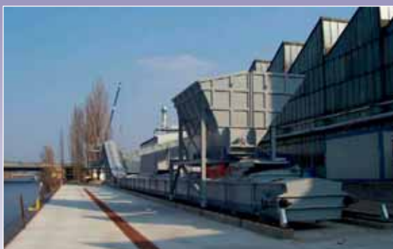
Conveying systems at the harbor
