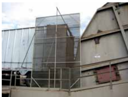
DustTamer Wind Screen side panels prevent cross wind dust generation at tippler to hopper transfer point.
