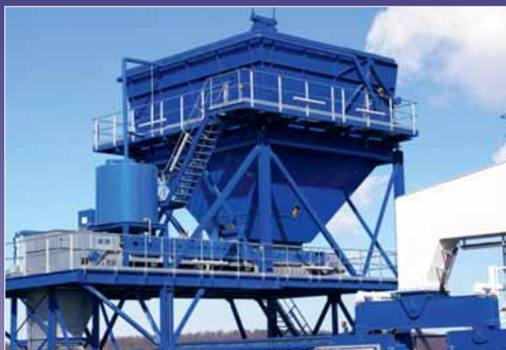
Hopper cars for ship unloading
