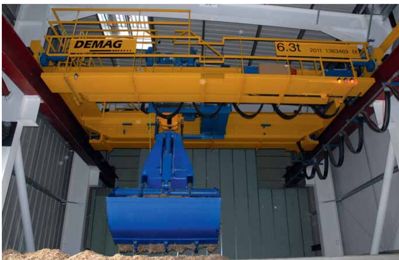
Demag Cranes' fully automated crane system at Sky's CCHP plant.
