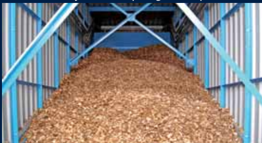
Wood chip intake for a brewery steam boiler
