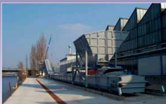
Conveying systems at the harbor
