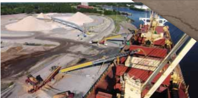
ONE MACHINE LOADS, TRANSFERS AND STOCKPILES
