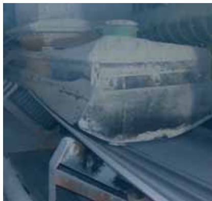
Prior to the upgrade, dust exited the back of the chute, fouling the tail pulley and affecting visibility.
