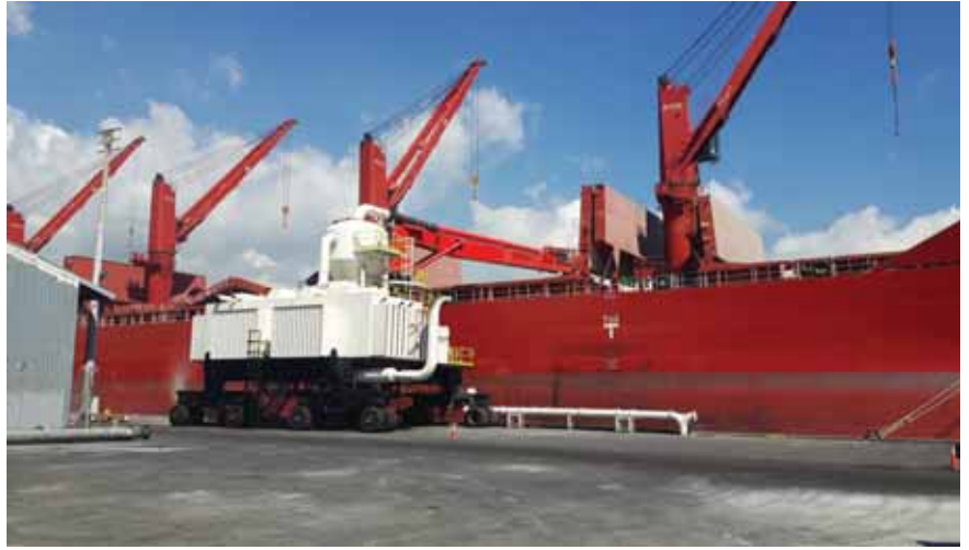
A Van Aalst ship unloader supplied to Lafarge Mauritius, conveying product through a removable pipeline on the dock which connects to pipeline running under the dock surface — keeping the dock free for other operations.
