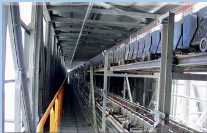
Clinker pan conveyor
