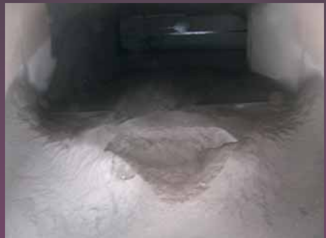
These 'before' photographs illustrate the extent of the blockages.
