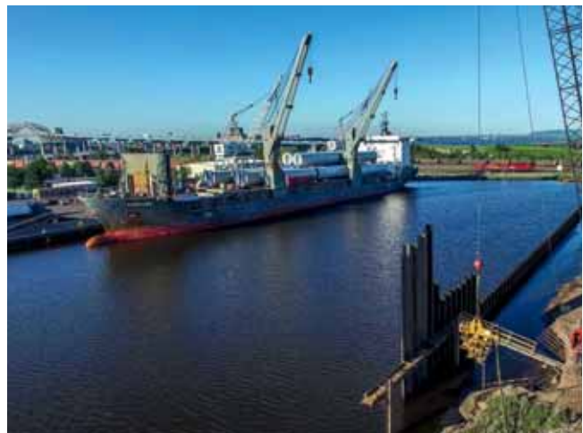
In the foreground, sheet pile is being driven along the Dock D section of the Port of Duluth Intermodal Project during summer 2015. The Fortune can be seen in the background, discharging wind turbine tower sections at the Port Authority's adjacent Clure Public Marine Terminal.
