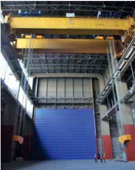
Broekman Project Services indoor warehouse facility, offering overhead crane capacity of max 700 tonnes.
