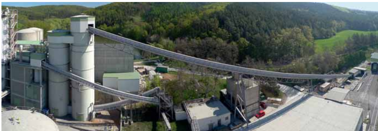
Tubular and U-shaped conveyor belt configurations.
