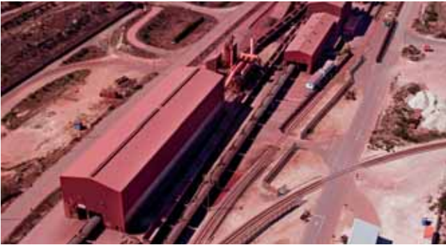
Trains and wagons entering the tippler at the Saldanha Iron Ore Terminal.
