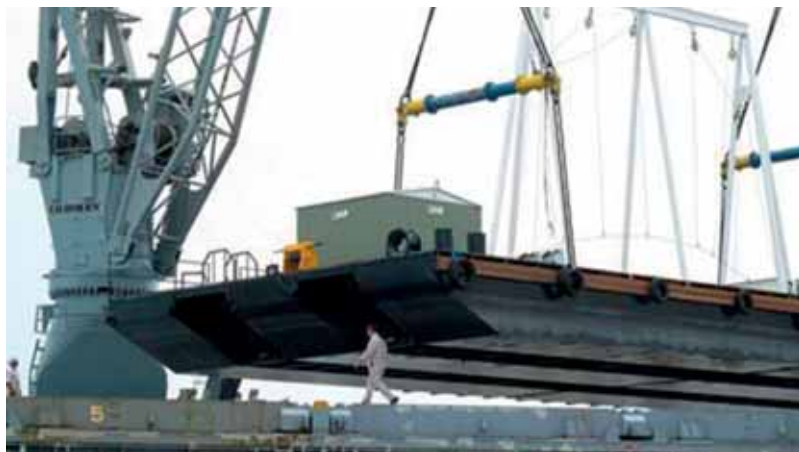
A 100-tonne barge being lifted in Port-la-Nouvelle.
