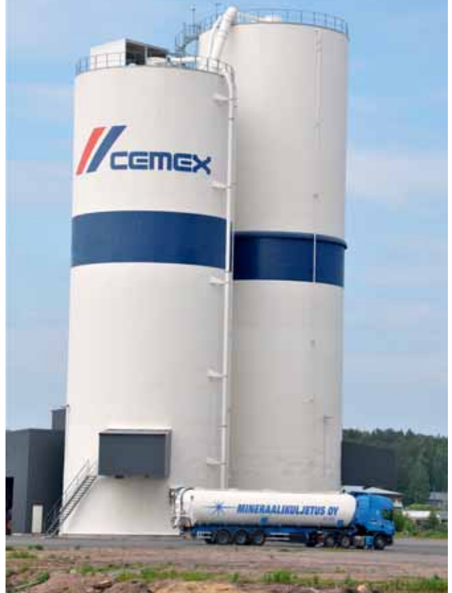
At the Port of Loviisa, cement is stored at two silos which belong to Cemex.
