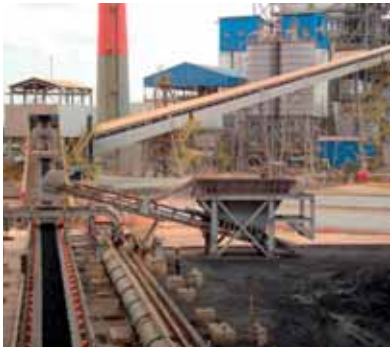
Coal complex in Itaqui, Brazil.
