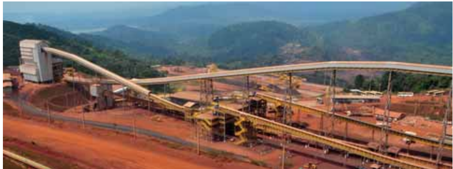
44 belt conveyors, with capacities ranging from 1,200tph to 10,800tph.
