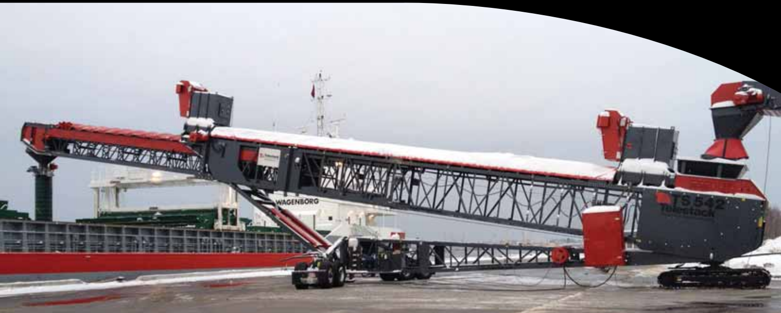
Mobile Radial Telescopic Shiploader loading fertiliser to coaster vessels from warehouse
