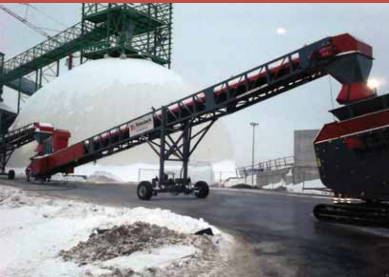
Mobile Links feeding Shiploader from warehouse
