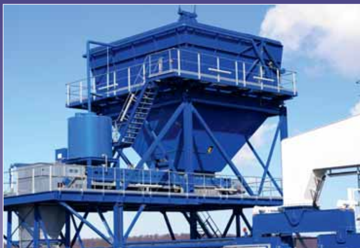
Hopper cars for ship unloading
