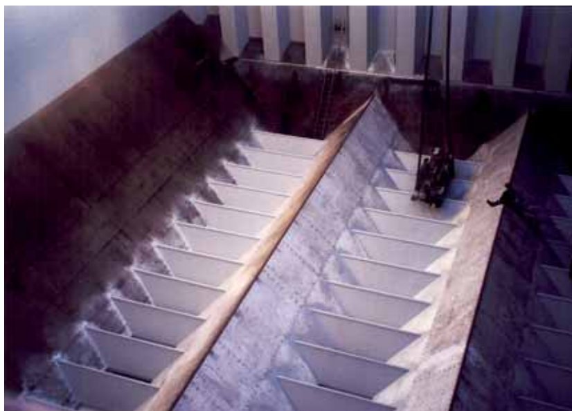
Installing an optimized lining system reduces the risk of spillages, their consequent environmental impact and clean up costs.
