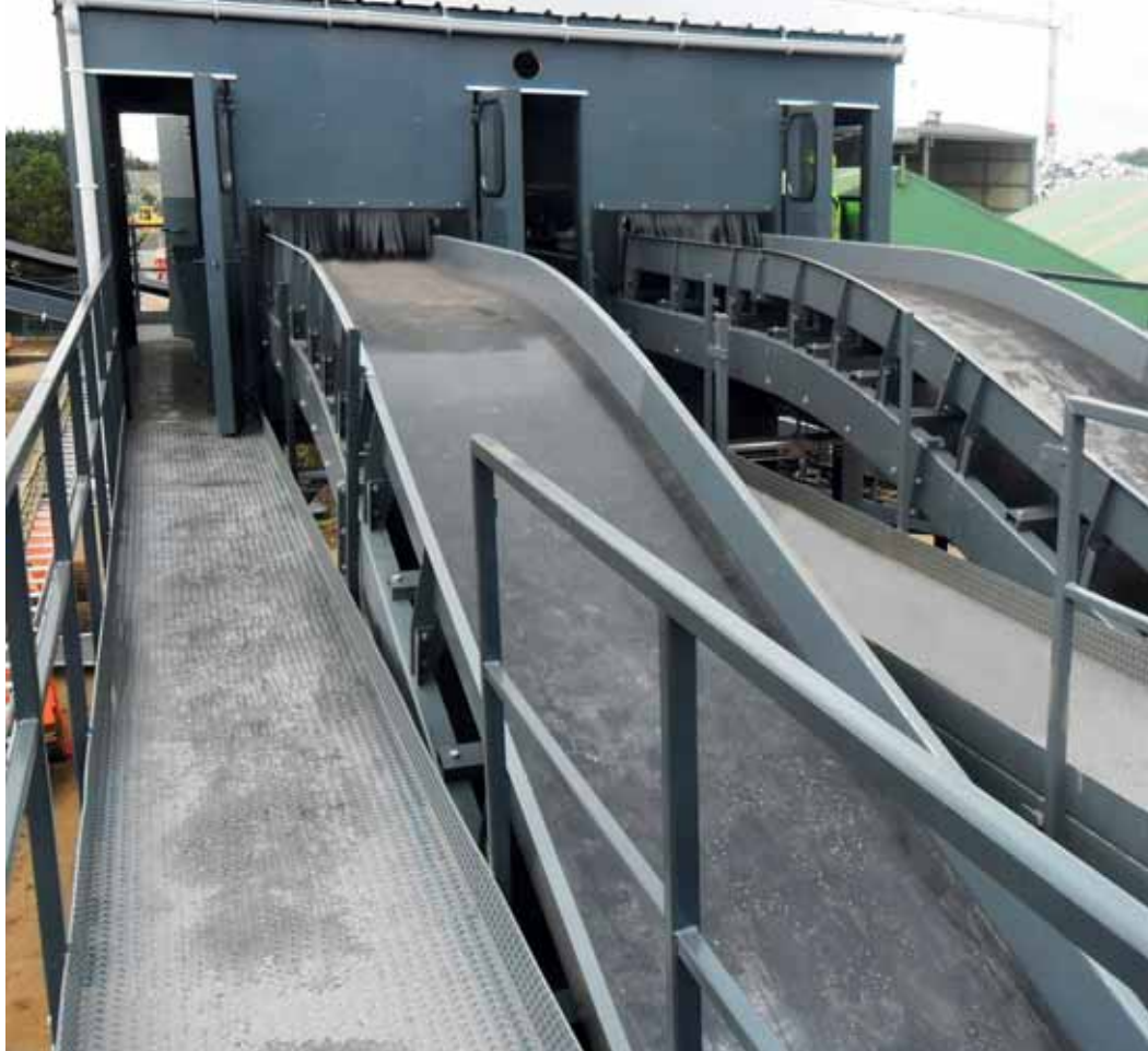
Part of a recycling sorting line that holds a various of conveyor belts and a sorting cabin.
