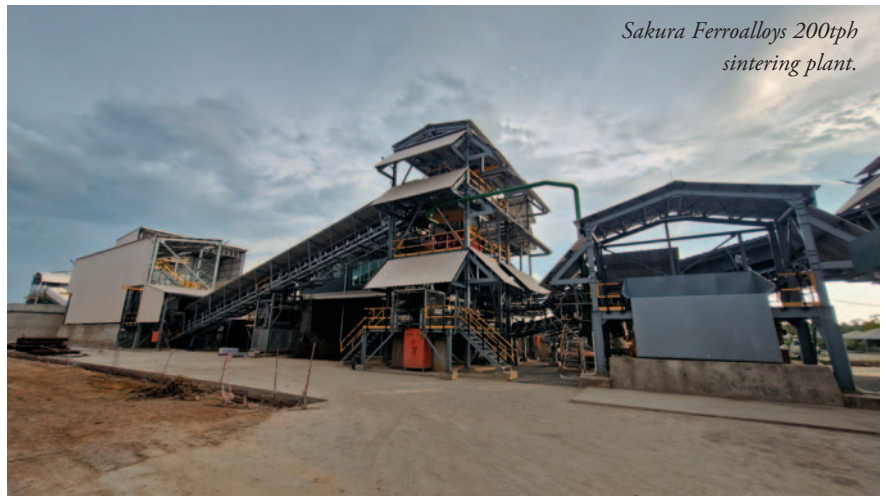
Conveyors under construction, forming part of the Sakura Ferroalloys plant, Malaysia.
