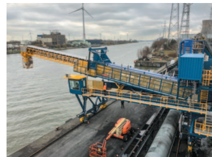
De Regt conveyor systems upgraded an existing tower structure with a diverter valve, new conveyor and a mobile shiploader.
