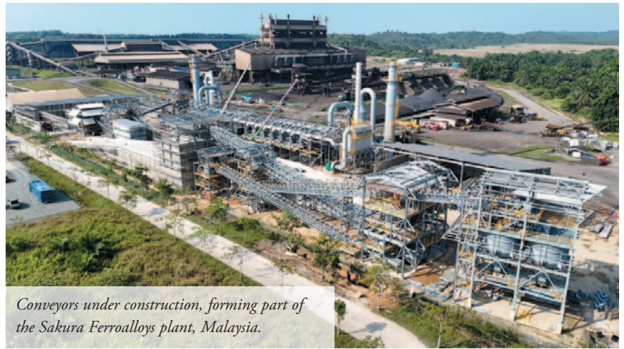
Sakura Ferroalloys 200tph sintering plant.
