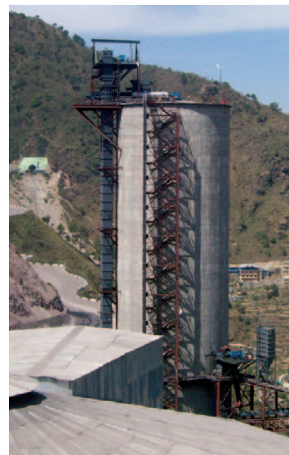
TSUBAKI NBC-K Bucket Elevator/Positive Discharge Type (right).
