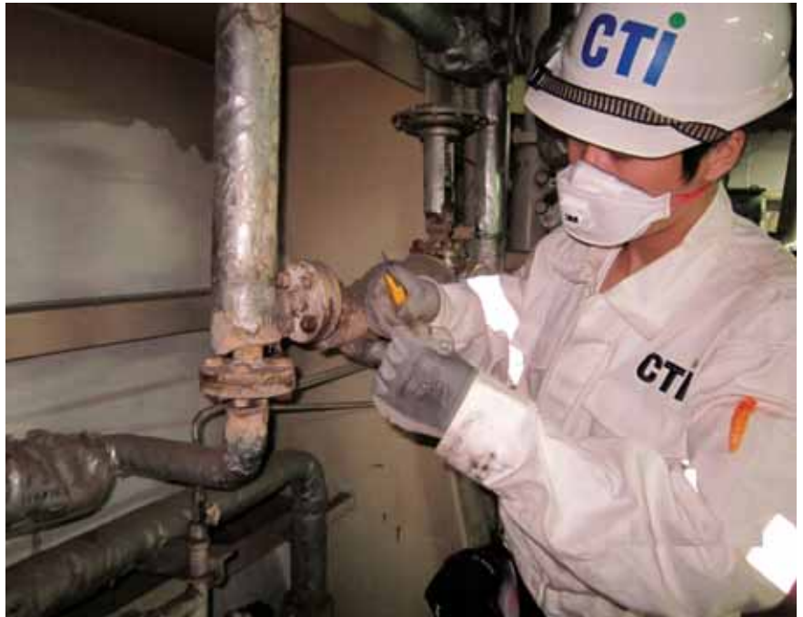
A CTI technician collecting asbestos (above) and hazardous material (below) samples.
