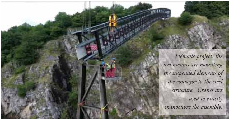
Project Flémalle: the line runs across country, over steep rocks. The pipe conveyor navigates easily over these inclines and gradients.
