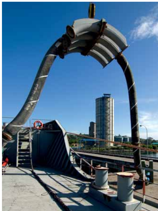
Fig. 5: Ship-to-shore pipeline connection.
