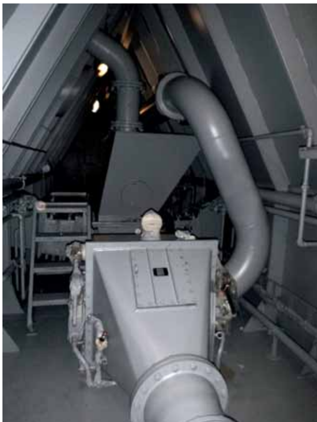
Fig. 4: IBAU Screw pump for cement carriers.
