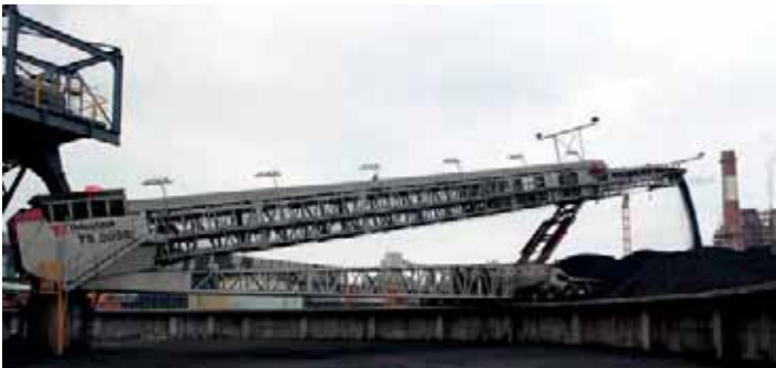
Radial telescopic stockpiling coal @ 2000tph in powerplant receiving from ship unloading system
