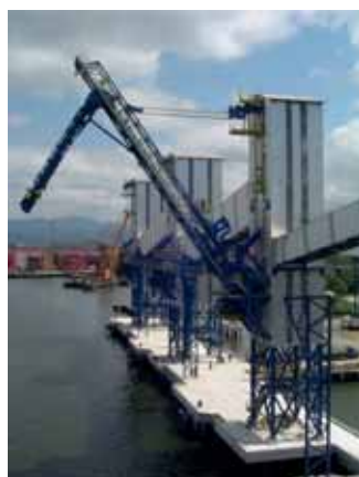
Fixed steel tower.
