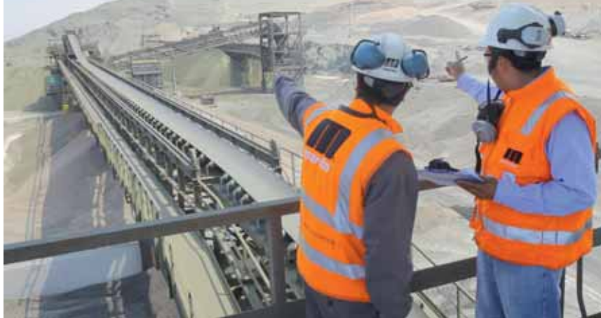
By taking responsibility for routine maintenance and inspection, technicians help customers maintain system performance, while minimizing unplanned shutdowns.
