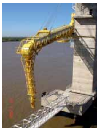
Fixed concrete tower
