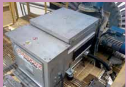
Successful installation of TFO enclosure to a previous reel (box to the left with sticker)
