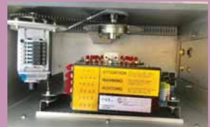
TFO inside enclosure
