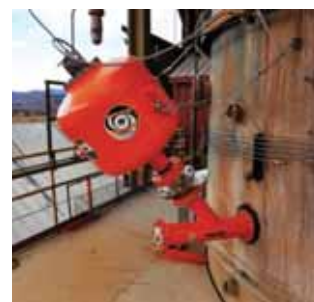
Martin® Core Gate technology allows air cannons to be installed and serviced without a process shutdown.
