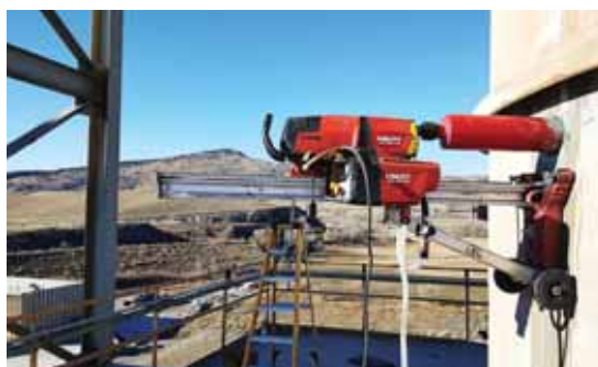
The drill cuts through outer wall and refractory, then retracts automatically.
