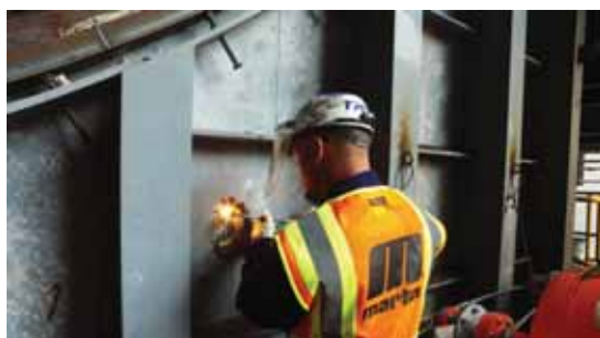
Technicians drill through the outer wall, then weld the Core Gate in place.
