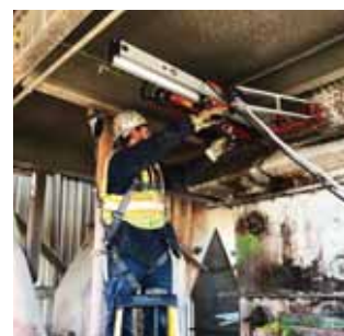
The core drill is mounted and aligned.
