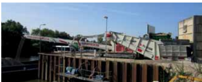
Mobile truck unloader (track mounted) loading barge directly from trucks and wheel loaders.
