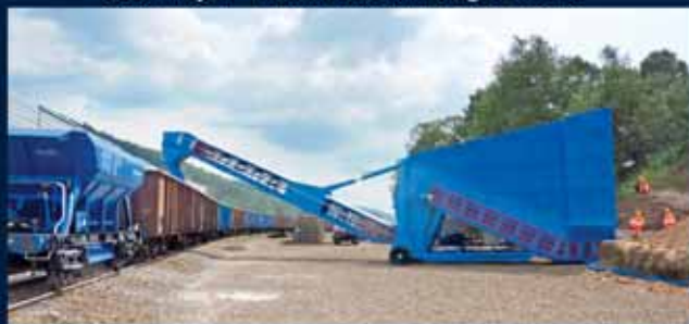
Mobile Stormajor™ loading to rail wagons
