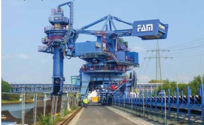
Fig 4: FAM CONTI ship-unloader CSU1100.14S, for use with vessels up to 2,500dwt, handling coal at a rate of 1,100tph, in Germany.
