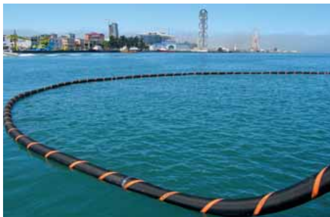
In the Batumi terminal in Georgia, highly resistant bunkering hoses from Continental transport fuel oil, carburettor fuels, and hot asphalt to and from the ships. Photo: ContiTech
