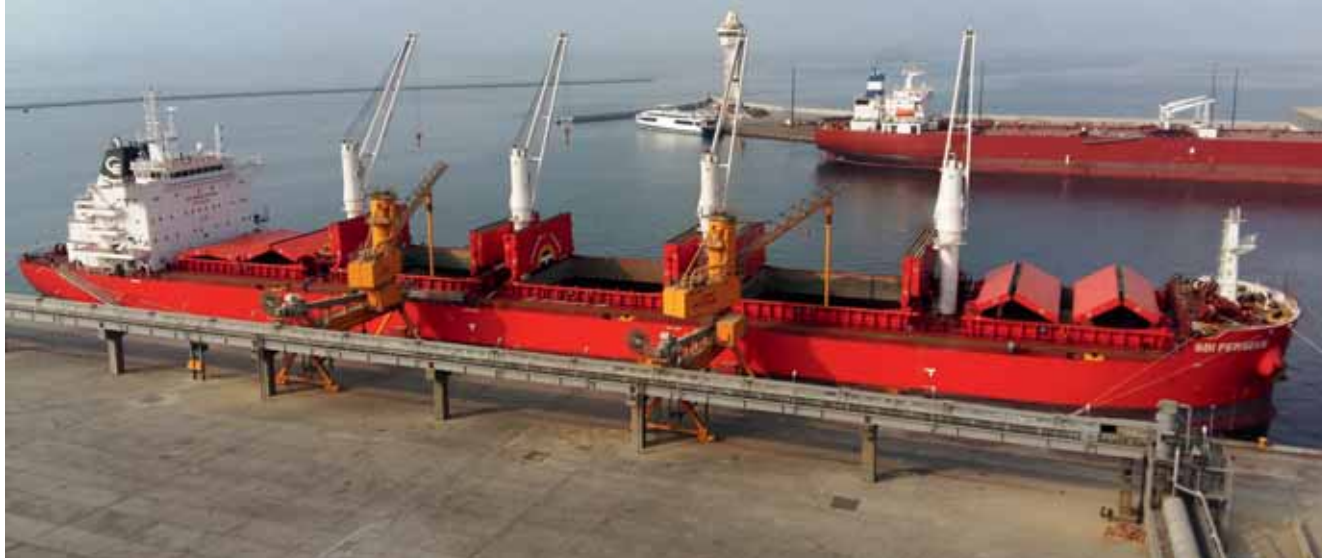
Two 600tph NIVs installed in Jazan.
