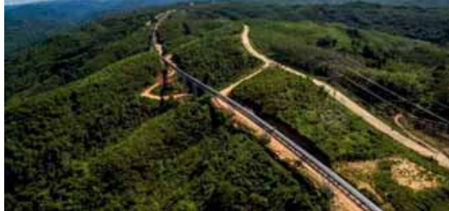
The route of the overland conveyor for the end customer, Cemindo Gemilang, passes through the middle of the rain forest.
