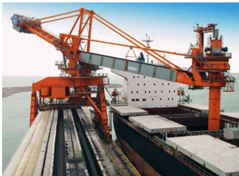
TK's high performance CSU, similar to that to be installed at Baolihua's Jiahuan Power Plant, in unloading operation at Huilai Power Plant, China.
