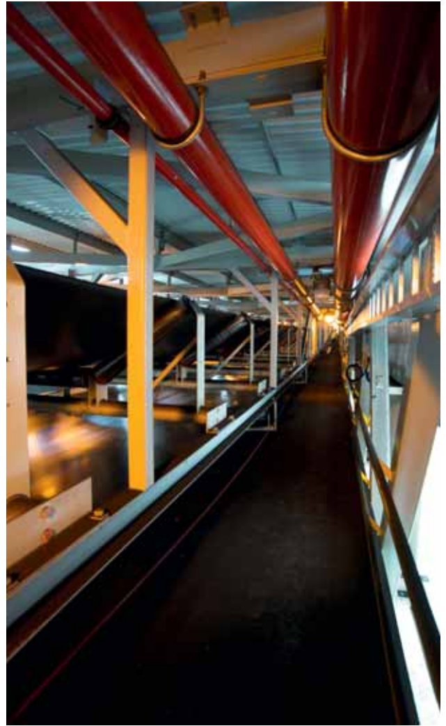
ContiTech conveyor belts are also in use during the interim storage on the platform. (Photo: ContiTech)
