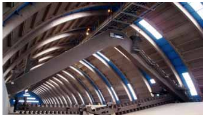
Pic. 4 Portal scraper reclaimers installed at Jaorf Lasfar.
