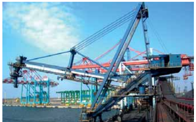
Picture 1.7: One of three ThyssenKrupp shiploaders built for TIS Terminal in Odessa, Ukraine
