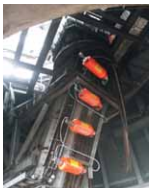
Picture 2: transfer chute.
