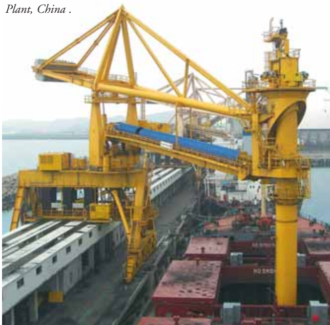
Picture 2.2 : ThyssenKrupp's 3 units CSU, similar to those to be installed at Zhujiang , in unloading operation at Huayang Power Plant, China .
