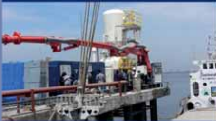
Jetty Mounted Ship Unloader
