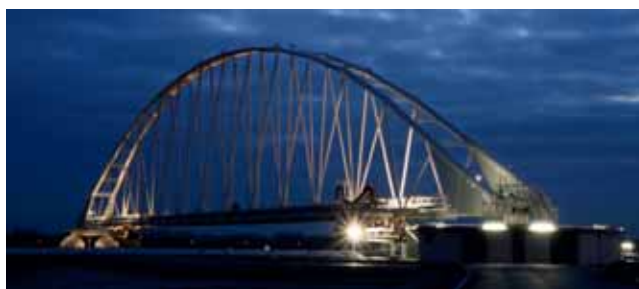
This sludge treatment system at the Port of Antwerp uses the world’s largest plastic energy chain, the E4.350. The project won the silver vector award in 2012. (source: igus GmbH)
