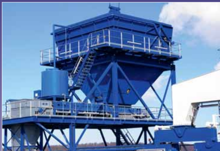
Hopper cars for ship unloading
