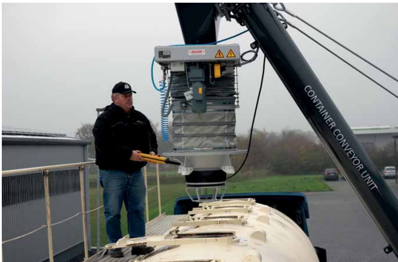
Fig. 5. Closed loading system with integrated filter unit for loading of graphite and coke in closed silo trucks.
