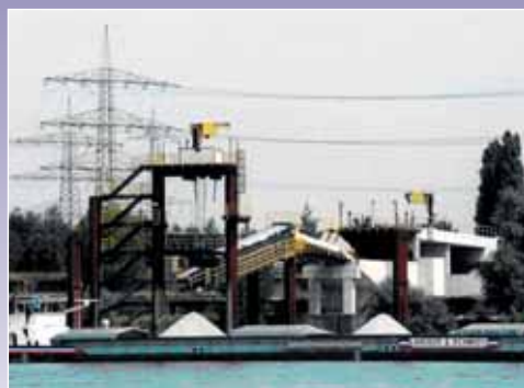
Ship loading systems
