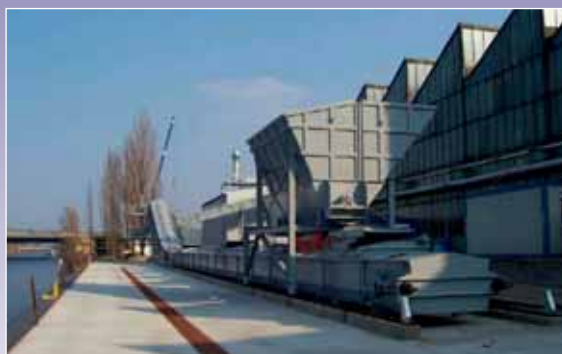
Conveying systems at the harbor
