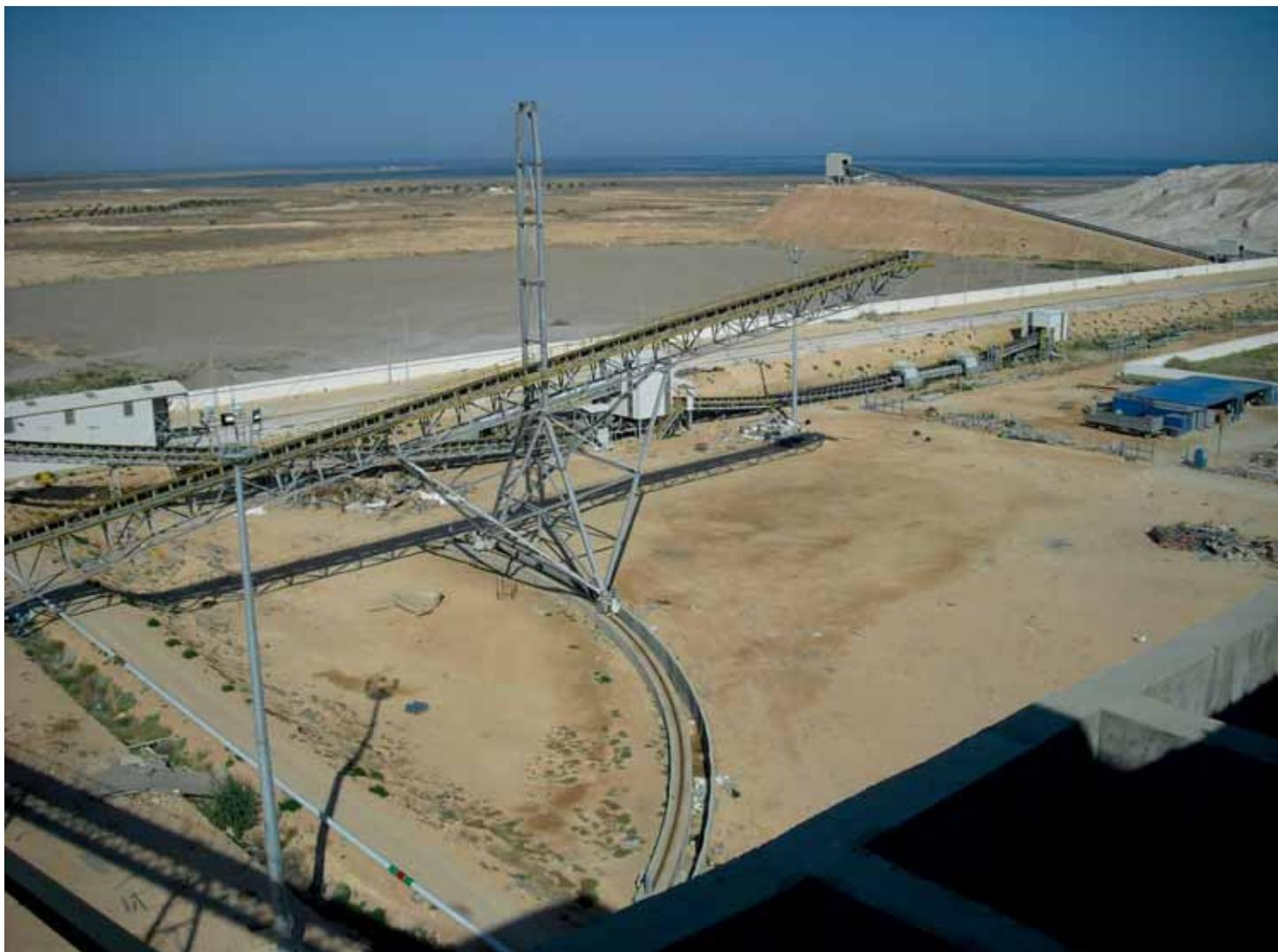
TAIM WESER has designed and supplied a dual phosphate conveying circuit for the TIFERT (Tunisian Indian Fertilizers) phosphoric acid production plant located in Skhira, in Southern Tunisia.
