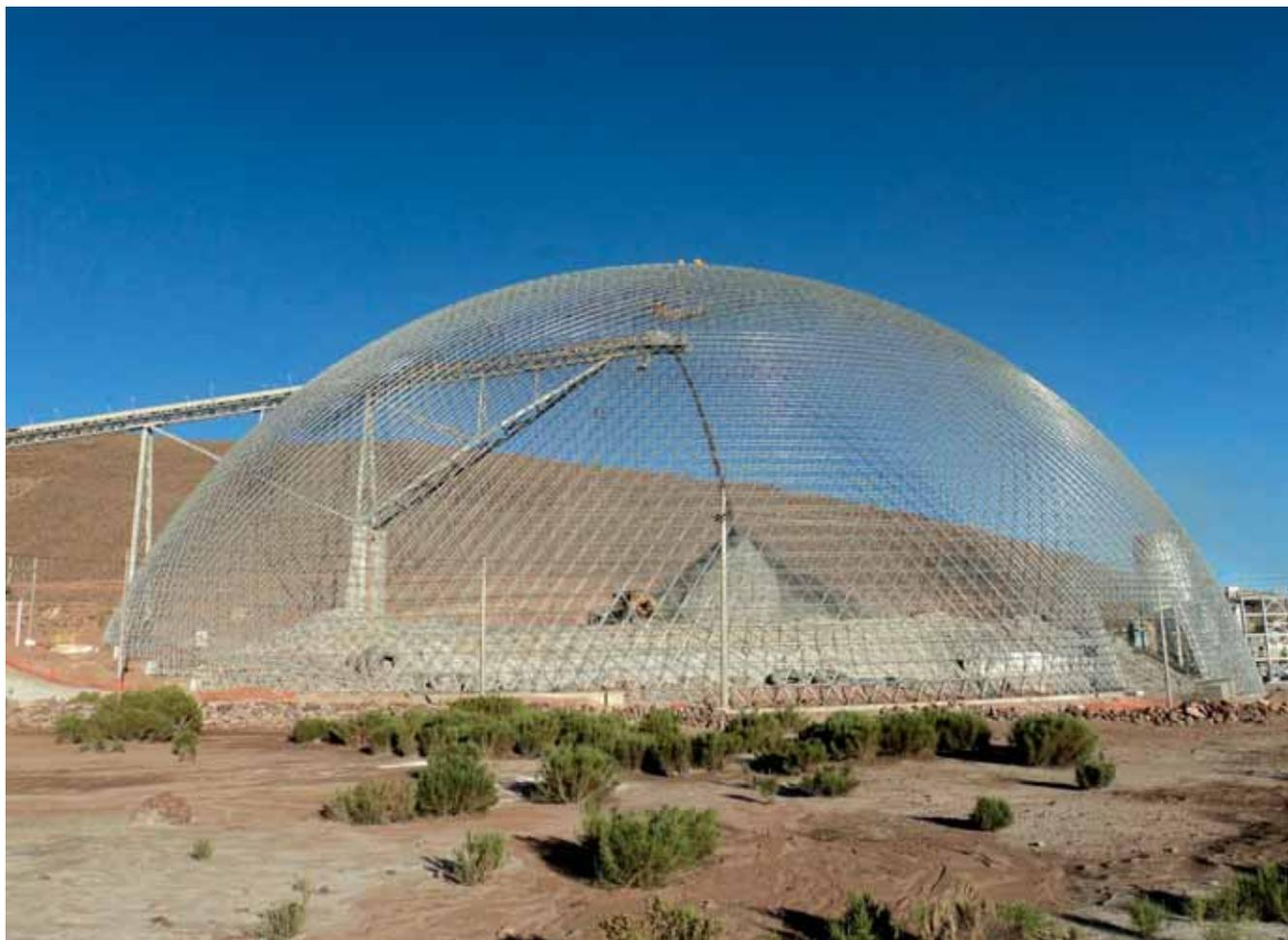
manufactured and supplied the dome. Key factors in the decision to employ a Geometrica dome solution for the site included the team's extensive experience, the capability to build around an operating stockpile, and the capability to follow an irregular shape for the supports.
