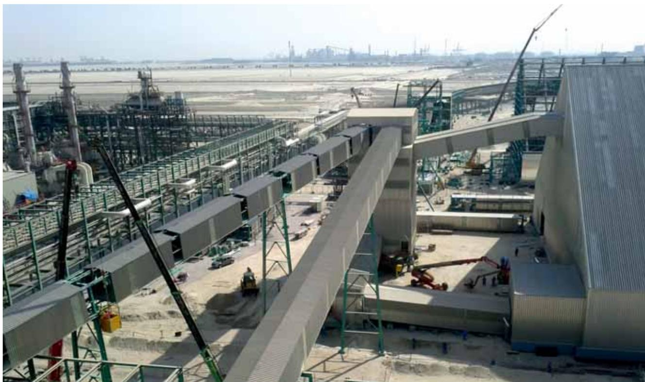
*Outgoing conveyor system and pipe conveyor in Qafco V and VI with storage hall (in far distance the TKF pipe conveyor running up to silo buildings of Qatar Aluminium Smelter).*
