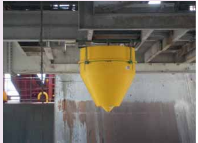
Figure 1: This is the initial height the hopper was installed prior to loading the first truck.
