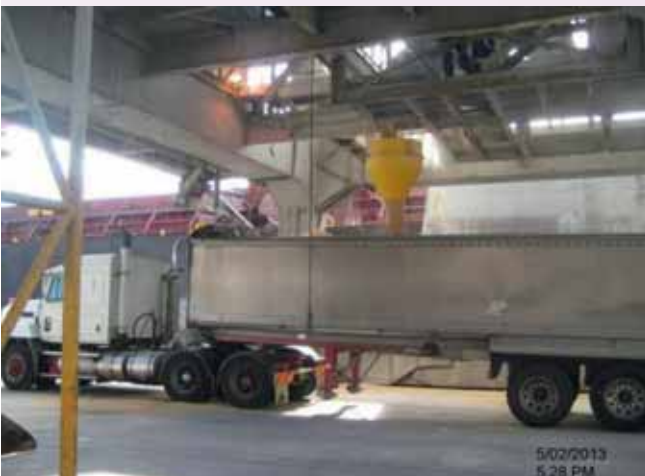
Figure 4: Unloader A DSH Hopper in operation loading a truck after further adjustments.
