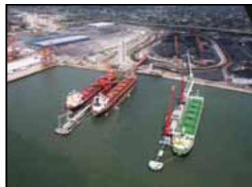
Pier IX Terminal
