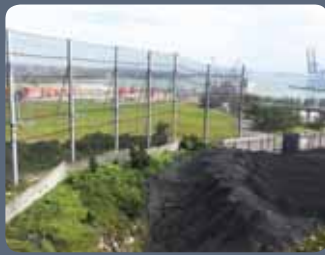
32m high fence for mountainside port storage
