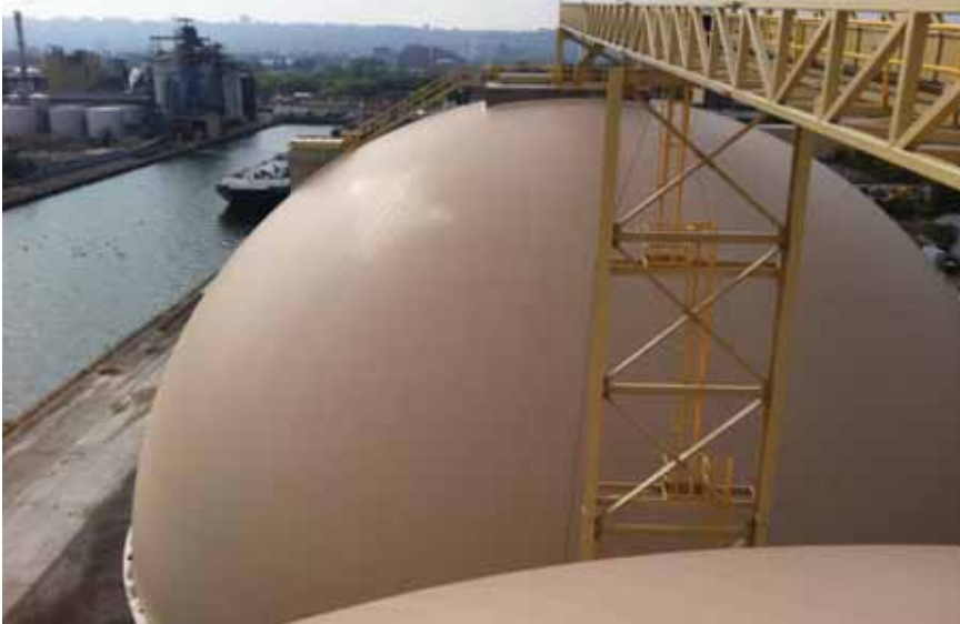
Grain domes built by Dome Technology for Parrish & Heimbecker in Hamilton, Ontario, Canada.
