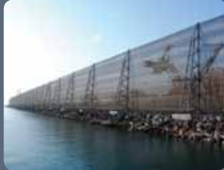
1.5km fence in marine environment
