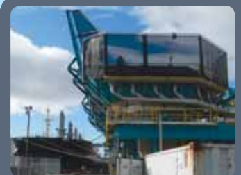
Hopper fence in conjunction with fog system
