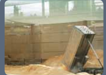
Fence with roof for easily blown dust
