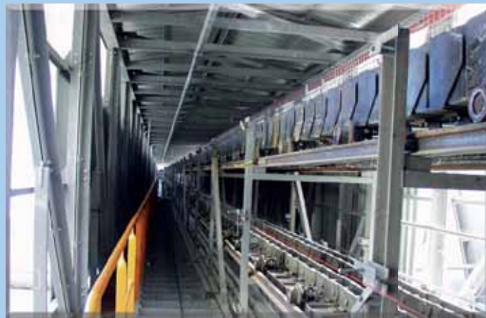
Clinker pan conveyor
